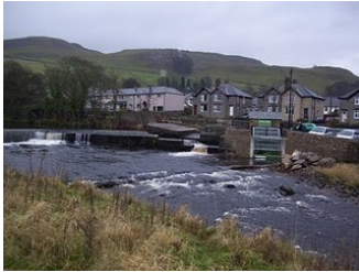
The wear at Settle with the screw and generator house
