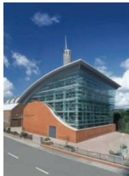
Pulrose Power Station Is there a 'greener' way of meeting our energy needs?
